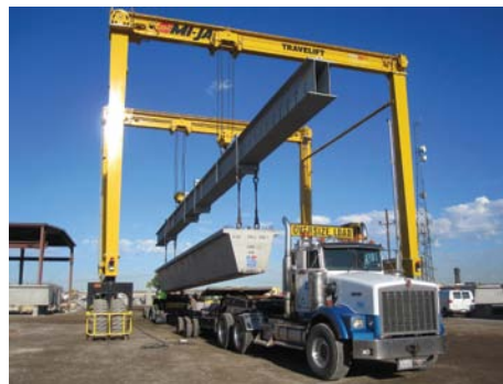
Prestressed U-Beam being loaded in USCPG's local plant for transportation to Sky Harbor.
