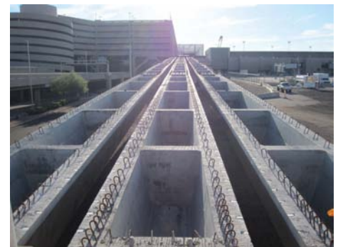
Top side view of typical U-Beams erected at Sky Harbor.
