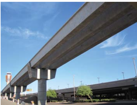
Prestressed, Concrete U-Beams rising toward Sky Harbor's Terminal 4 Station.
